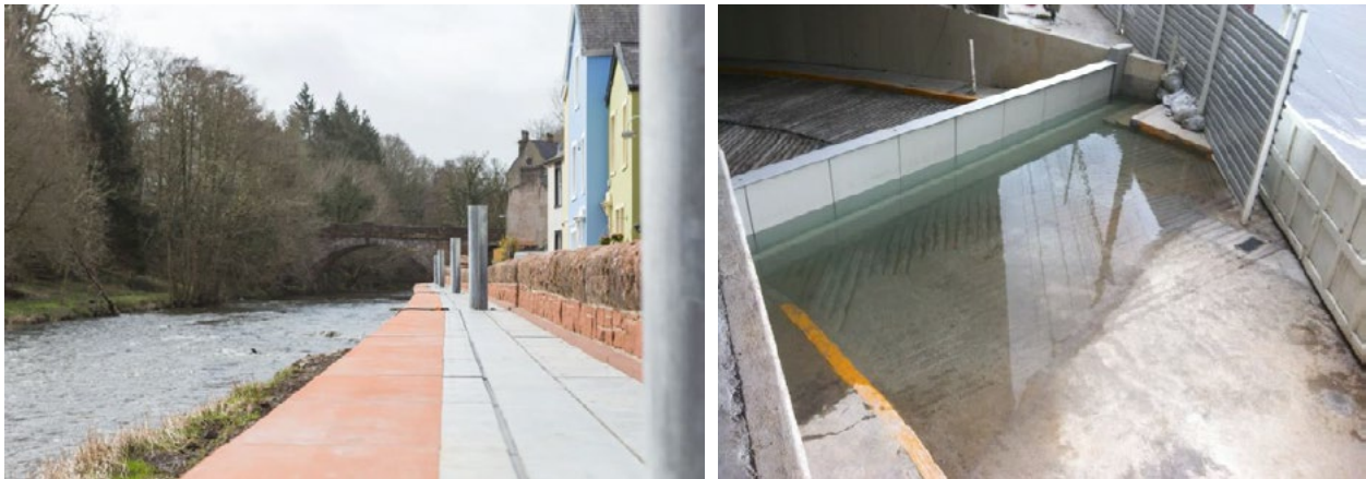
PHOTO 5 (left) | SAFB as a flood wall in Cockermouth, England. The recessed wall provides additional height to the town's flood wall in case of high water and access to the waterfront during normal conditions.
