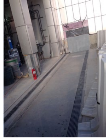
PHOTO 3 (left) | Protecting Lourdes hospital in Binghamton, NY. Arrows show areas with FloodBreak gates installed.
