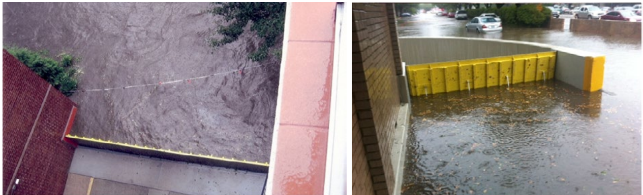
PHOTO 1 (left) | FloodBreak protecting a vehicle entrance to an apartment building in Great Neck, NY.
